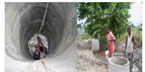
Well under construction at Kpayou Town, Margibi County
